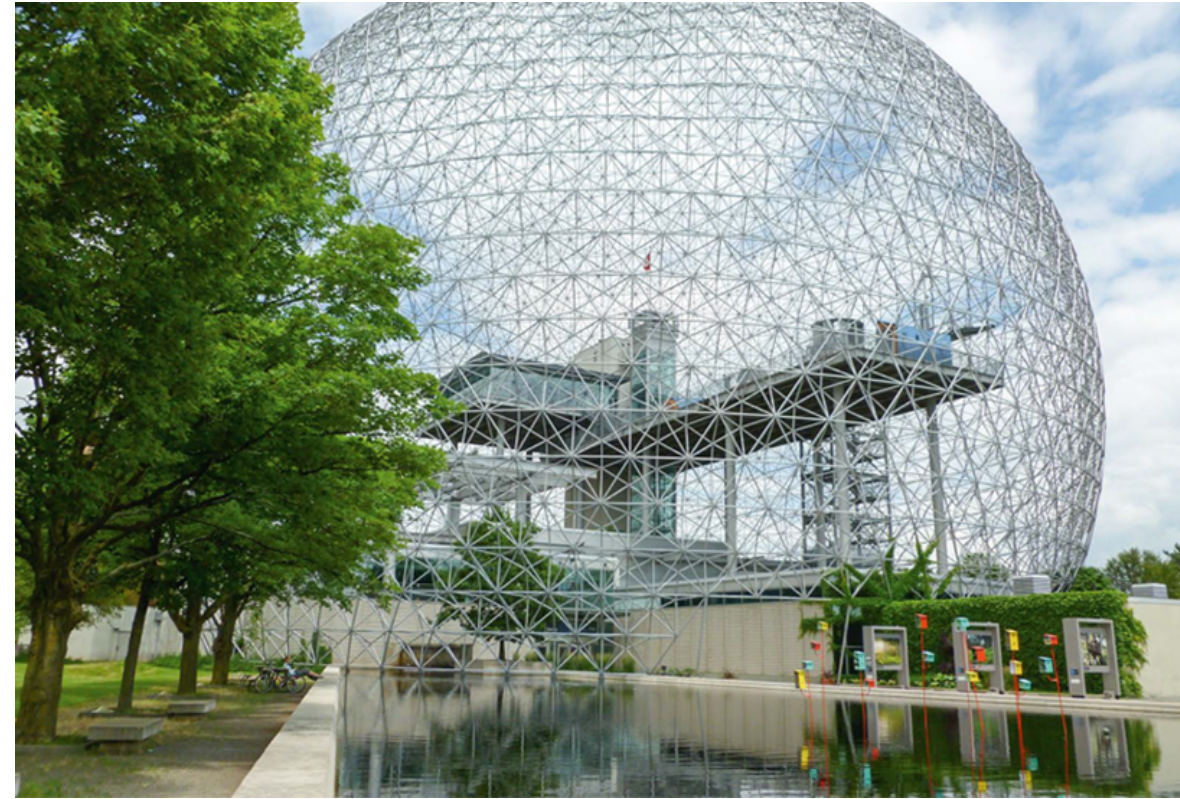
Exhibition pavilion "Expo-67" in Montreal (height 62 m, diameter 76 m).
