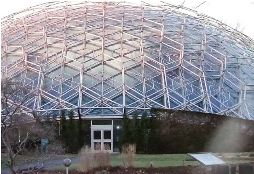
St. Louis, USA. The dome "Climatron", used as a greenhouse of the botanical garden (height 21 m, diameter 53 m). Made in aluminum structures. 1960 year
